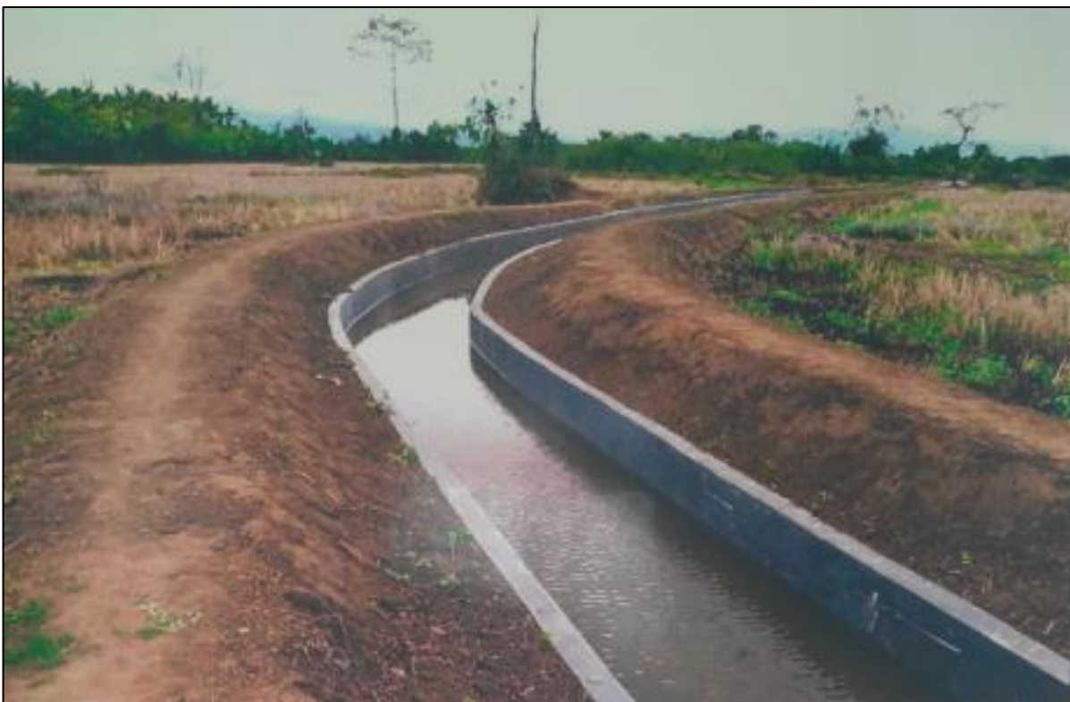
Irrigation Structures in Changlang district of Arunachal Pradesh
